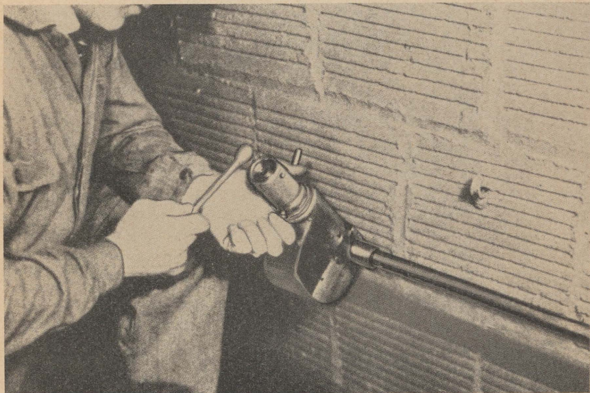
PLATE 104.—Velocity power pipe bonding press.
