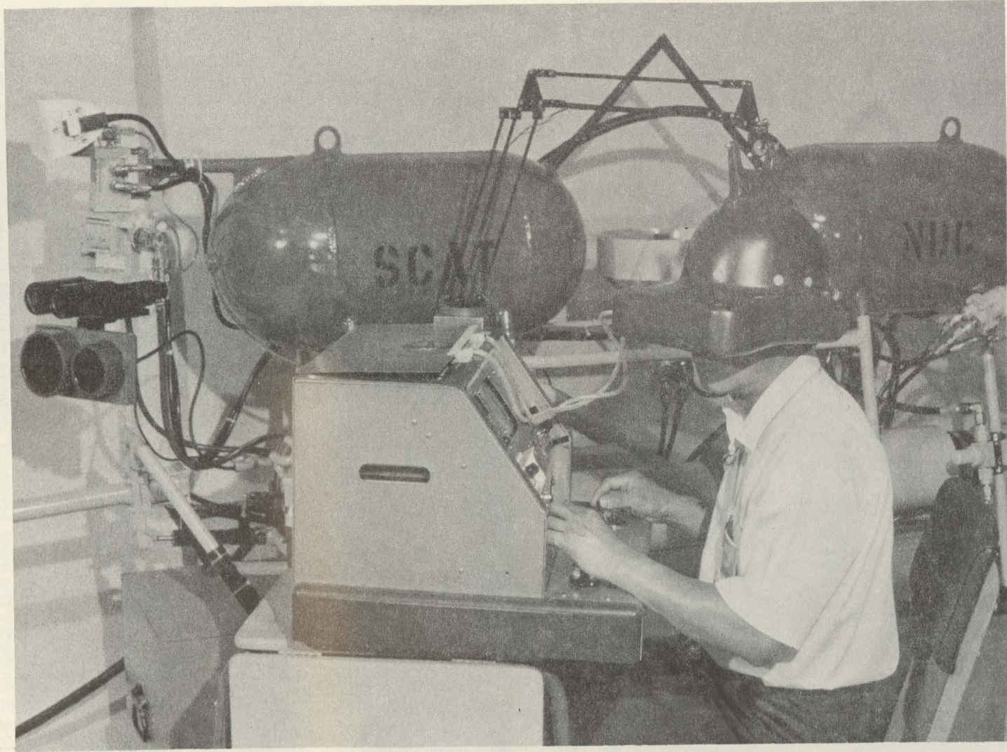
Figure 8. Head-coupled stereo TV was tested extensively on SCAT . Though cumbersome, the system showed conclusively that head-following camera orientation should be incorporated into undersea work systems. 244-1-73
