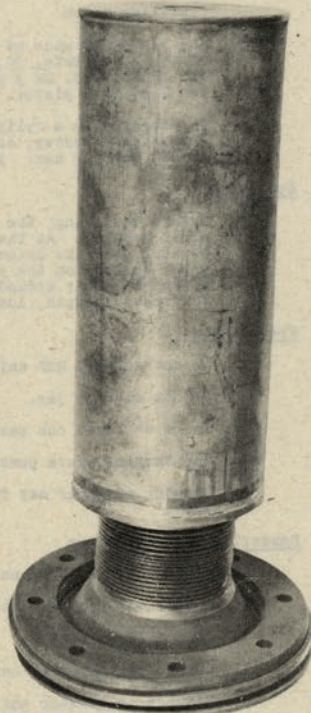
Fig. 6 - Depth Charge Booster Extender and Booster
