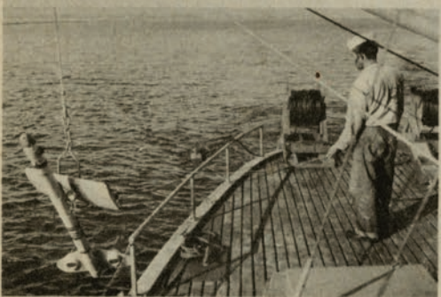
3. PUT BUOY OVERSIDE AND LOWER DETECTOR INTO WATER
