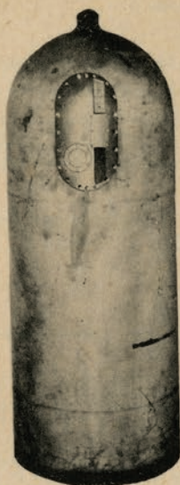
Fig. 12-- Mk. 13 Warhead With Mk. 4-1 Pistol
