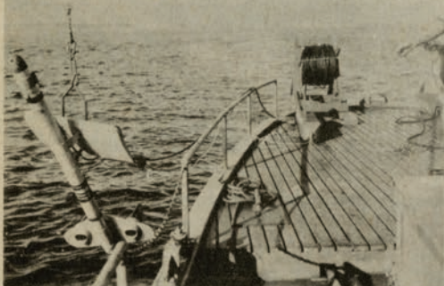
2. ATTACH AUXILIARY BRIDLE TO HOIST WITH PELICAN HOOK
